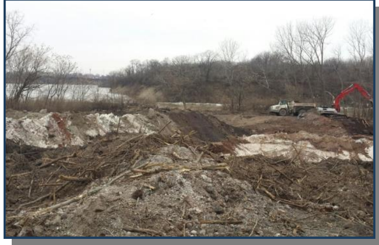
Steel mill slag removal
