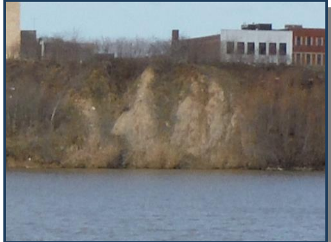
Stream banks at the sites are nearly vertical and highly eroded.
