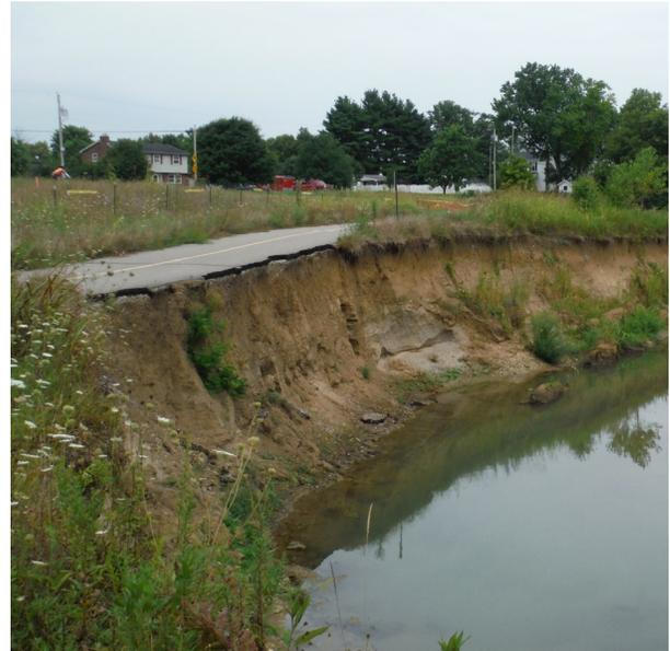
*Dry Fork Creek streambank. Note area of active erosion and failing bike path pavement.*
