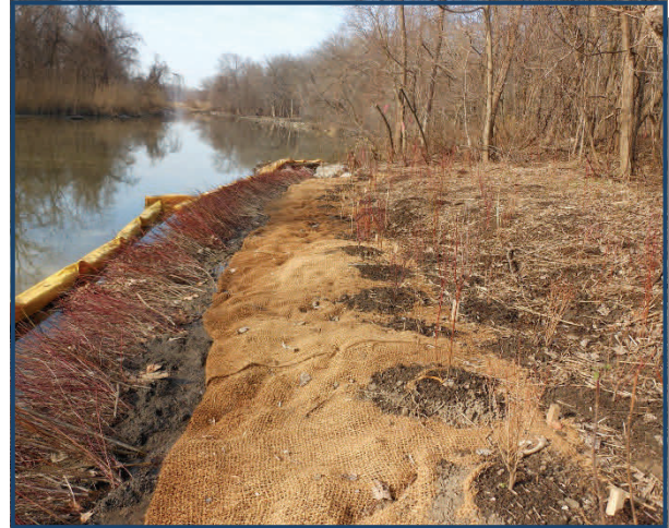
Natural bank stabilization included installation of branch layers and native shrubs.
